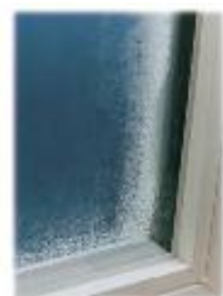
Traditional Box-Shaped Spacer Heat transfer through traditional box-shaped spacers, used to separate glass layers, can increase heat loss and cause condensation to form on the edge of the glass.
